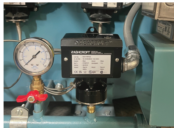
Oil pressure switch
