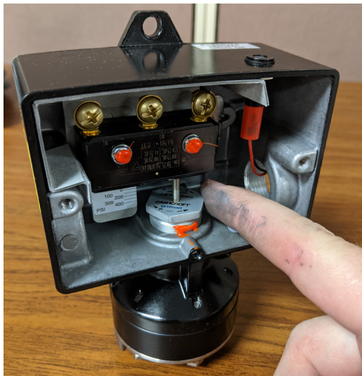
Gas or Oil pressure switch adjustment – Type B
