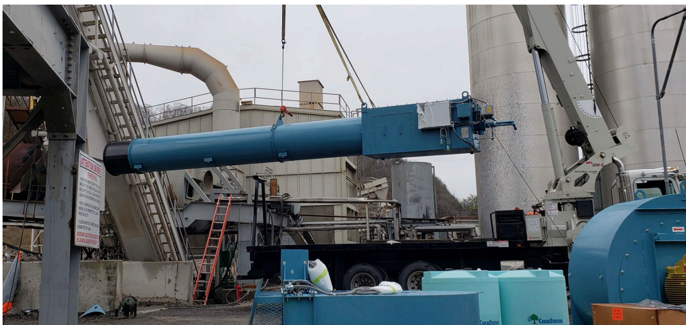
Installation of the Webster long nose burner, March 2020
