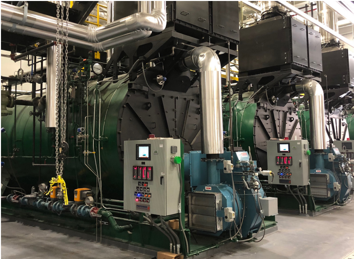
FDA's Johnstone boilers with Webster dual fuel JBEX burners.
