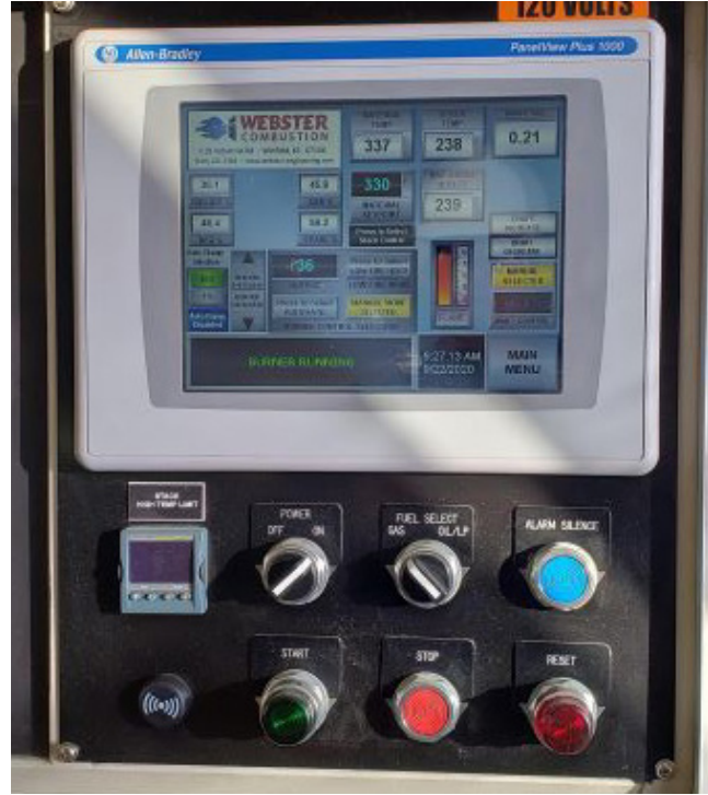
Before the controls retrofit (left), and after (right), showing the new Webster Combustion ABMS (Asphalt Burner Management System), with PLC-based functionality and a modern HMI.
