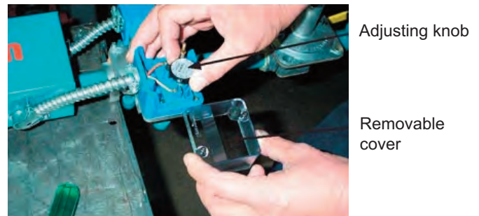
Figure E-4 Gas Pressure Switch Adjustment
