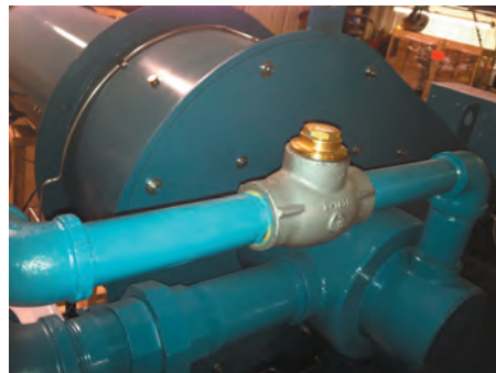
Figure B-14.1 Center Gas Balancing Valve
