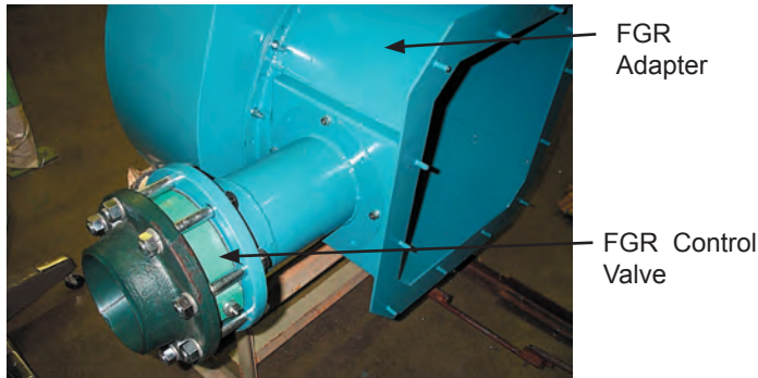
Figure B-23 FGR Control Valve
