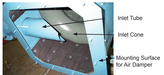
Figure B-22 FGR Inlet Tube
