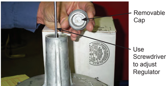
Figure E – 9 Main Gas Pressure Regulator Adjustment
