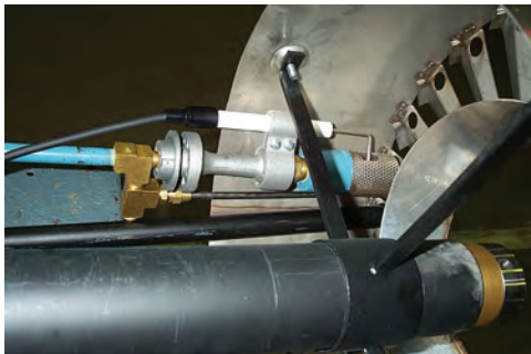
Figure B-11 Pilot and Scanner Sight Tube
