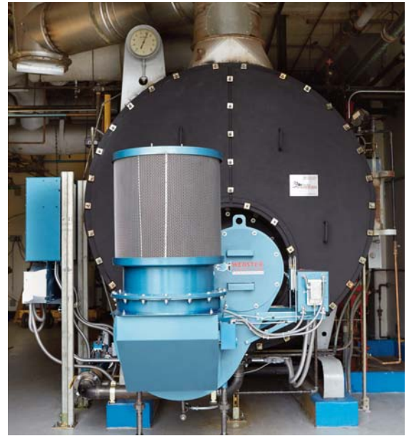
HDFX BURNER INSTALLATION
